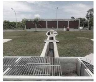
Picture 13: Inlet for connecting to faecal sludge carrying trucks
